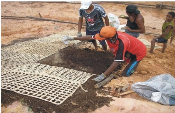
Fig. 10 Recuperation work in Sacavém Gully, São Luis Municipality, Maranhão State, Brazil, in February 2008, with the application of buriti geotextiles, manure and grass seeds (photo by José Fernando Rodrigues Bezerra).
