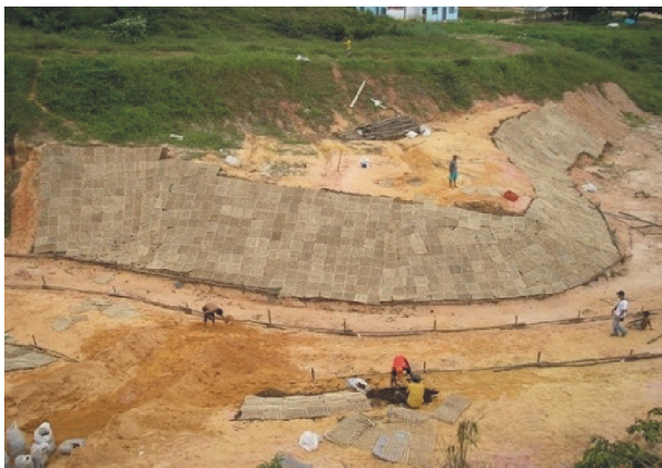
Fig. 11 Gully wall completely recuperated in Sacavém Gully, São Luis Municipality, Maranhão State, Brazil in February 2008, with the application of buriti geotextiles, grass seeds, manure and nitrogen, phosphorus and potassium fertilizers (photo by José Fernando Rodrigues Bezerra).
