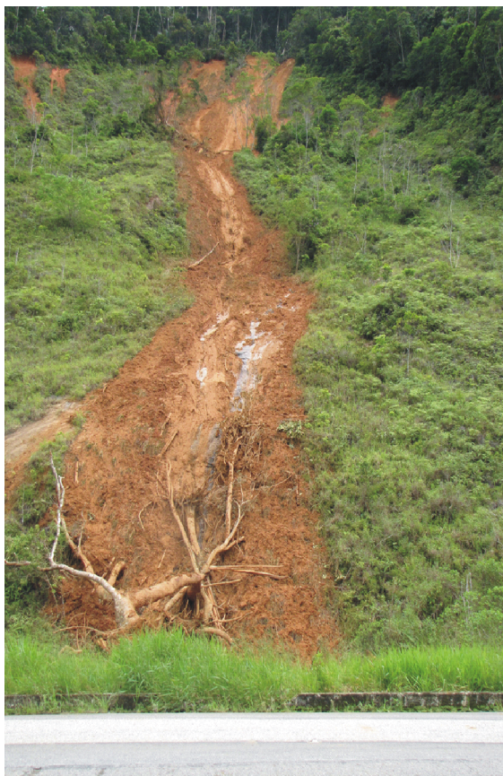
Fig. 3 Shallow landslide scar on Rio-Santos Highway, Ubatuba Municipality, São Paulo State, Brazil, in December 2009 (photo by Maria do Carmo Oliveira Jorge).
