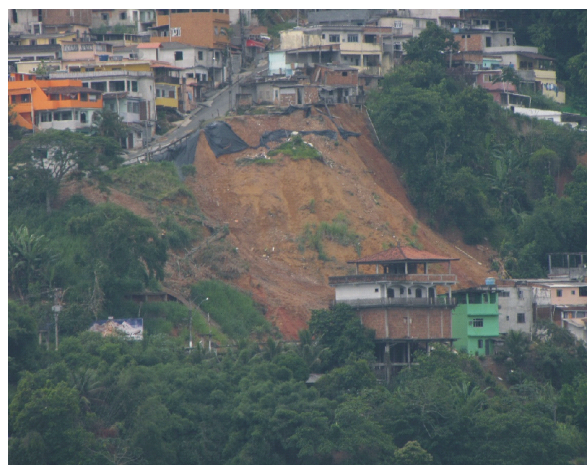
Fig. 4 Landslide scar in Angra dos Reis Municipality, São Paulo State, Brazil. Over 40 people died within the municipality due to landslides associated with about 200 mm of rain in 24 h in December 2009 (photo by Antonio Jose Teixeira Guerra).
