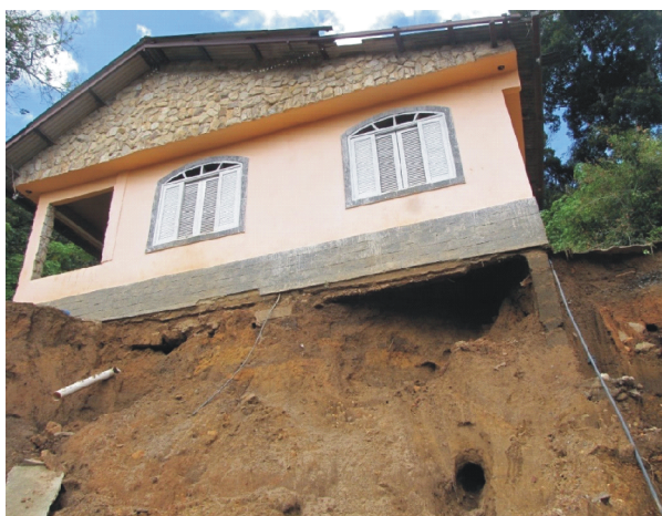
Fig. 1 A landslide scar formed due to heavy rainstorms in April 2013 in Petrópolis Municipality, Rio de Janeiro State, Brazil. The house was condemned on safety grounds (photo by Antonio Jose Teixeira Guerra).
